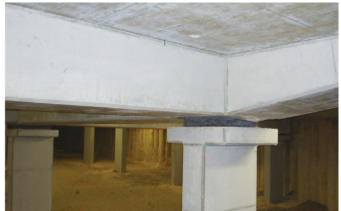
EXAMPLE OF COLUMN ISOLATION
