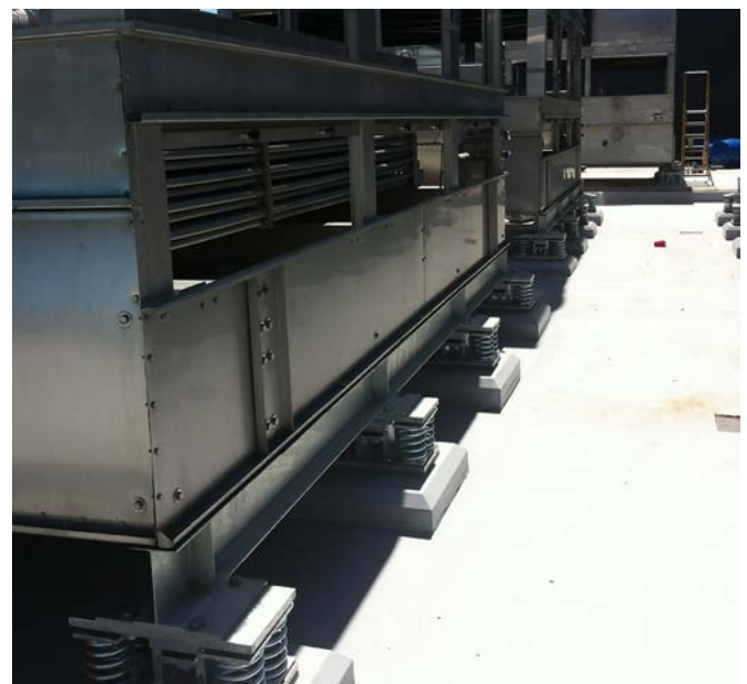
EXAMPLE OF SEISMIC ISOLATION
