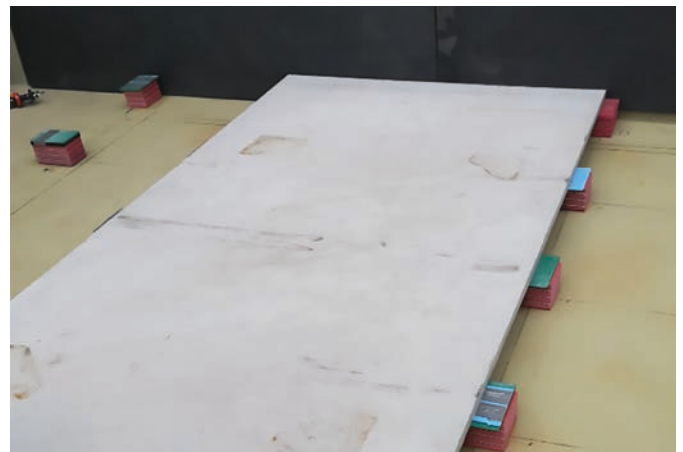
FC/CFC FORMWORK INSTALLATION EXAMPLE
