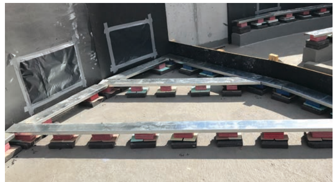
BEAM AND DECK INSTALLATION EXAMPLE
