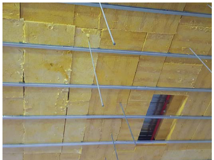
BARRIER CEILING INSTALLATION WITH INSULATION INFILL
